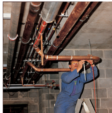
Hot Water Temperature Maint.
